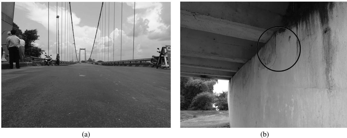
**Fig. 2.** Defects identified from previous visual inspection: (a) Road surface with abnormal shape where the middle deck is situated lower than the design. (b) Concrete crack at the cross beam imply possible movement of the main deck section
