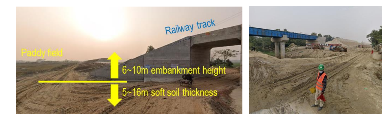
Fig2. Embankment constructions (google street view).
