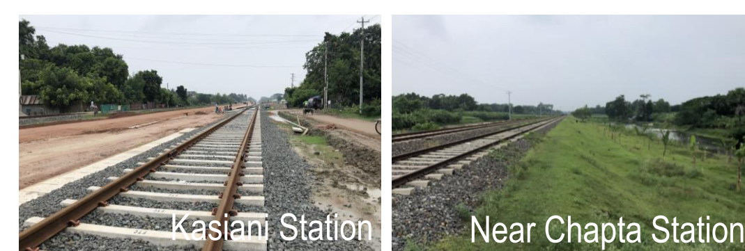
Fig5. Field visit to Kasiani and Chapta Station.
